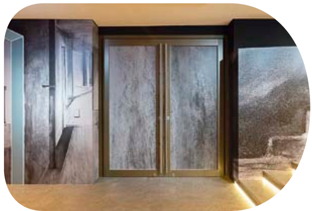
Fire-rated door with artistically designed film, integrated inside the IGU composition of Pilkington Pyrostop ®.
