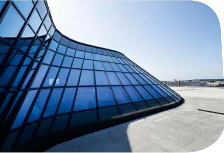
Faceted, sloping glass façade crown the roof. Pilkington Pyrostop ® 60-181 was used in the sloped glazing roof at the sides.
