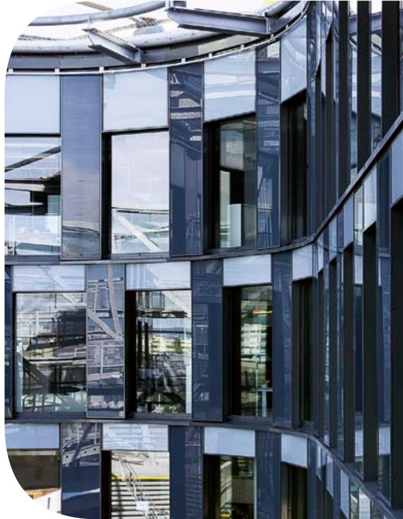
The inner façade in the core of the ÖAMTC building is designed for full protection against vertical flashover as a fire protection façade comprising Pilkington Pyrostop® insulating glass.
