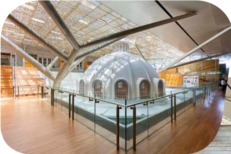
The tree-like support structure of the new steel-and-glass roof.
