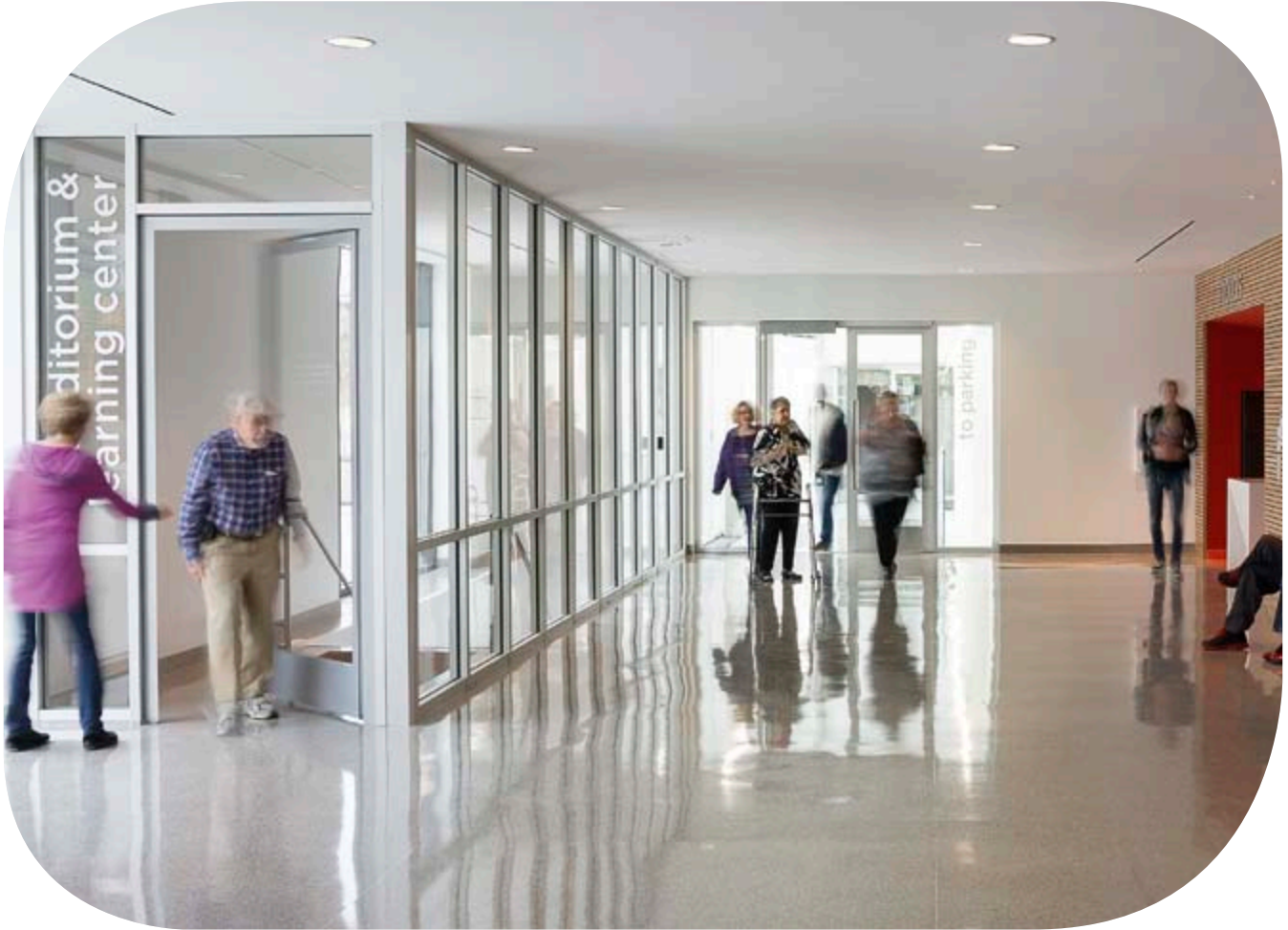
TGP's Fireframes® Aluminum Series partitions and Fireframes® Designer Series fire-rated doors with Pilkington Pyrostop ® in one of the egress staircases.
