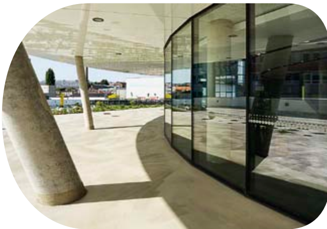
The façade system with Pilkington Pyrostop ® protects from a flashover to the escape and rescue routes located above.
