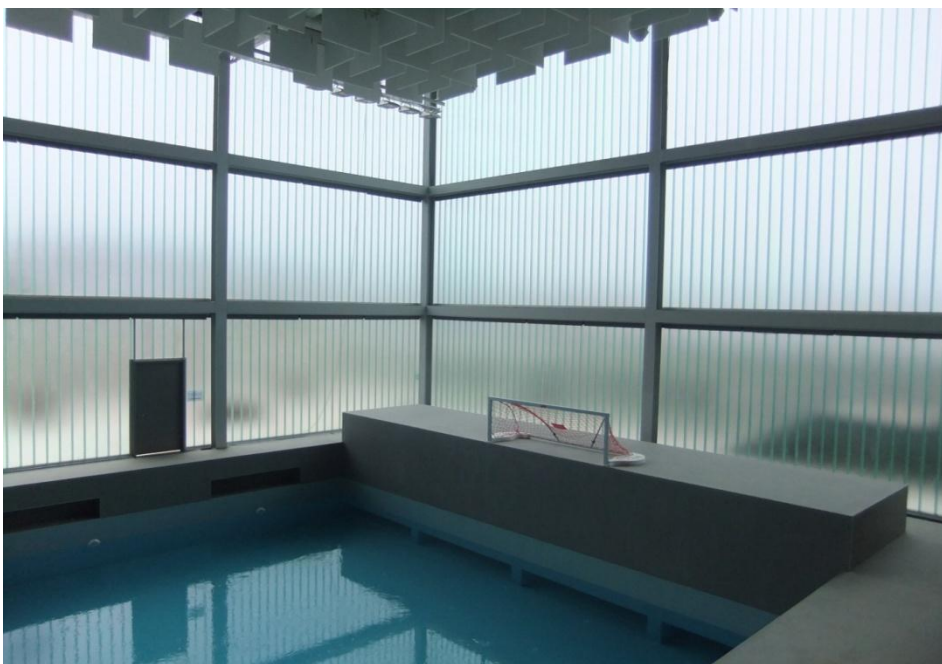
Picture 3: Comfortable natural daylight inside the nautical simulation and test basin building.
