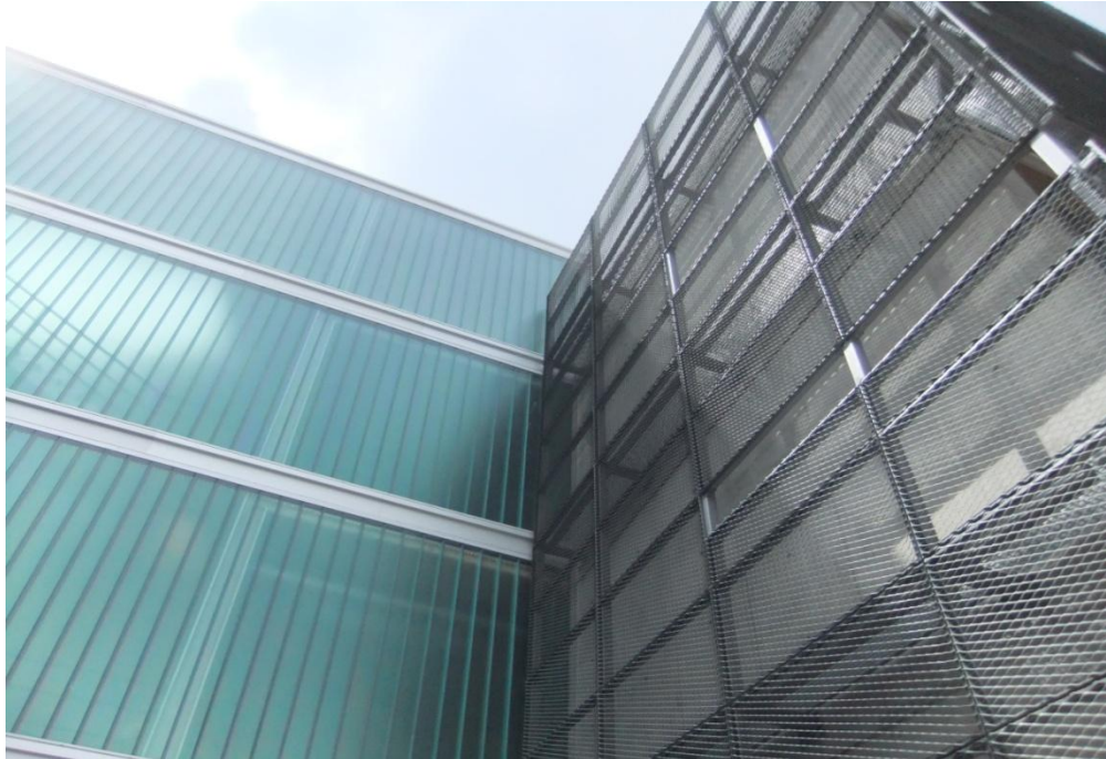
Picture 4: Combination of Pilkington Profilit™ with stainless steel and galvanized rib mesh
