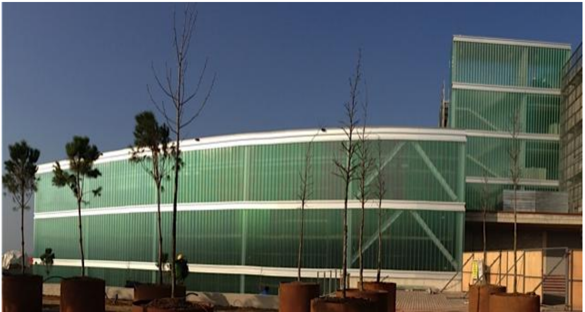
Picture 1: Nautical simulation and test basin building and staircases
