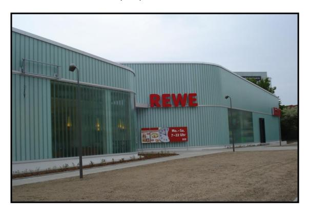
The design included double-shelled glazing with transparent thermal insulation (TiMax GL Plus F from company Wacotech GmbH), except in the shop window and clear glass areas. As such, the viewer sees an interchange of more or less transparent façade areas, whereby notably one of the main strengths of Pilkington **Profilit™**, namely its use as an option for curved and round elevations using glazing.
