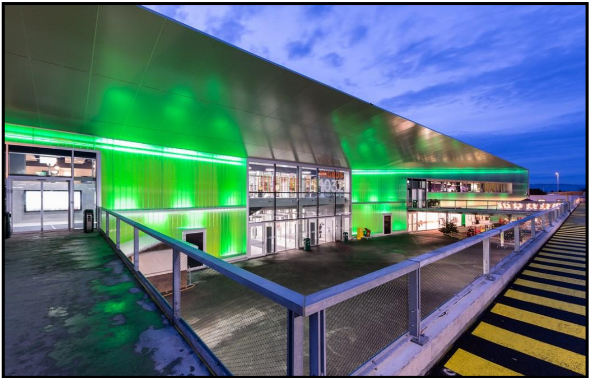
Lighting elements located between the wall and the glazing bathe the façade in a friendly, attractive light in the evening.
