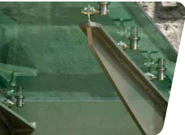
Seismic fittings in the **Planar™** | SentryGlas® Plus System installation: Alvarado Medical Centre, California
