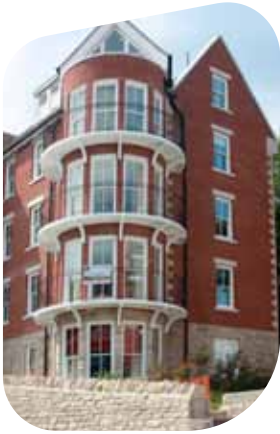
New construction of 7 flats and a penthouse Penlu, Swanage-Wales
