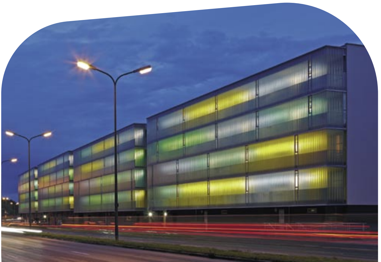
At night the facades on Innsbrucker Ring are a highly regarded illuminated object.
