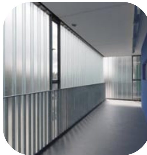
Natural daylight and effective noise protection for the entrance zones with a facade of Pilkington Profilit ™
