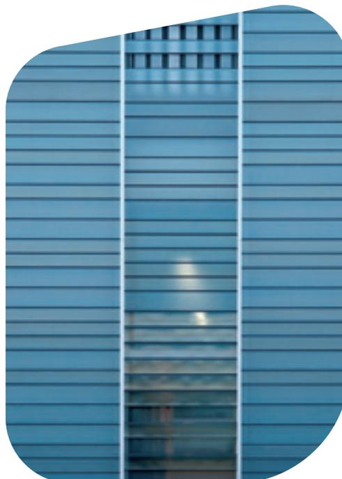
Installed horizontally: the façade shows variation in colour and structure via the use of Pilkington **Profilit**<sup>™</sup> in varying profile widths and finish types.
