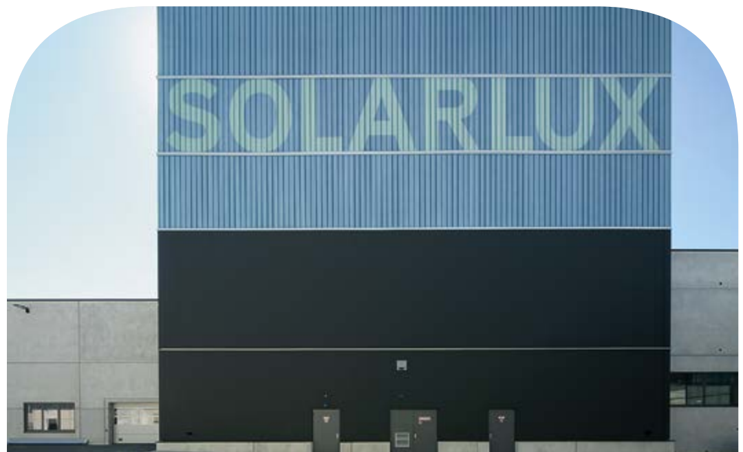
SOLARLUX Campus, Melle, Germany
