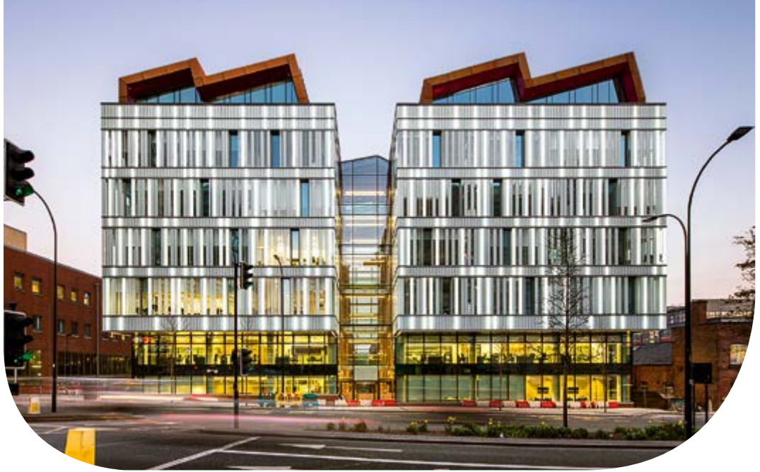
Sheffield Hallam University, Charles Street Building, Sheffield, UK
