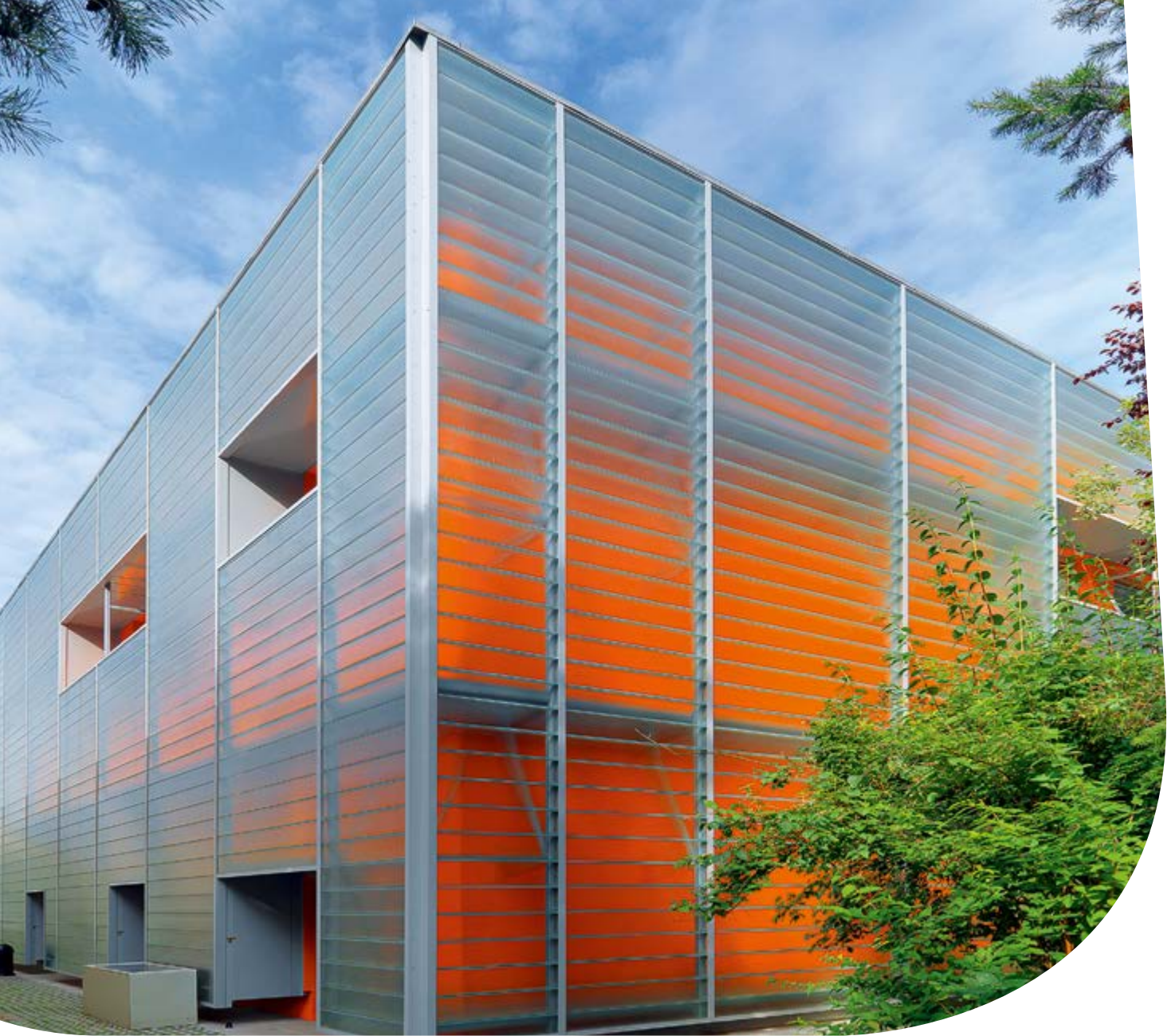
TECHNOPOLIS, Wrocław, Poland
