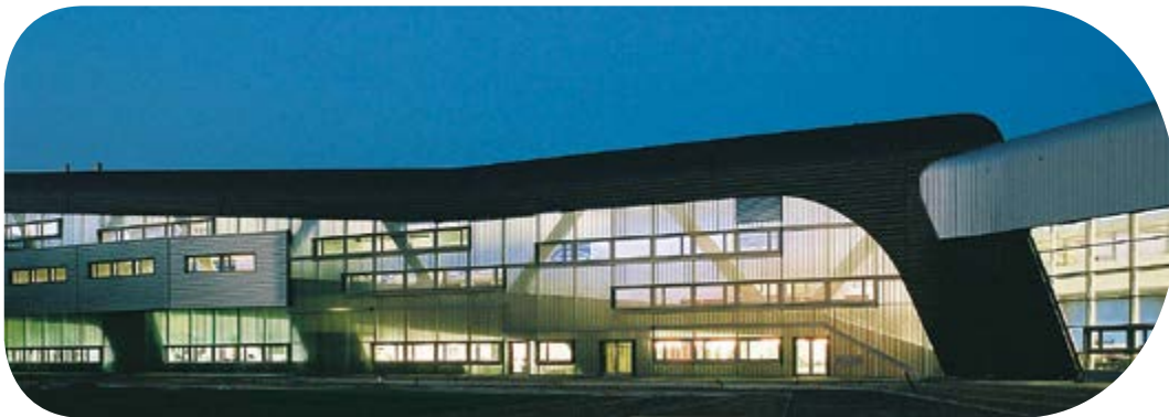
BMW AG Central Building, Leipzig, Germany Photography: Martin Klindtworth
