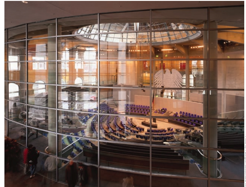
A stunning 16m high, flexibly suspended fire-resistant glazing protecting the plenary hall, German Parliament Building (Reichstag), Berlin, Germany.
