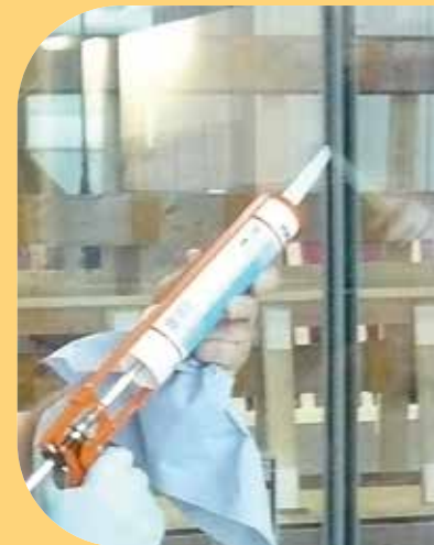
Glass is butt-jointed by means of applying suitable and approved silicone sealant in combination with ceramic fibre tape.
