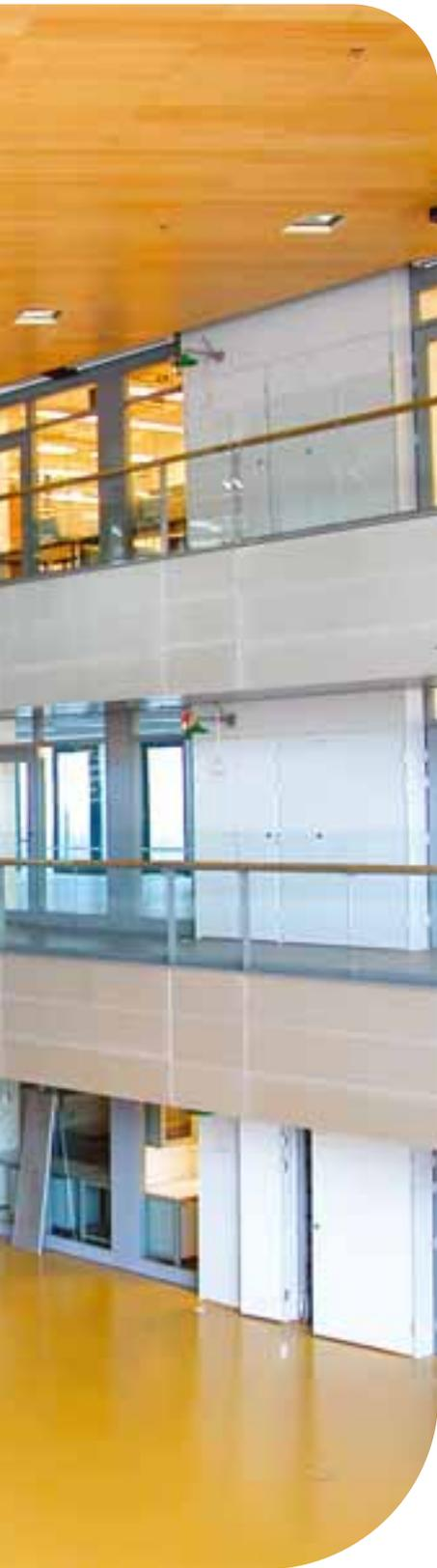
For the compartments, Pilkington **Pyrostop™** and Pilkington **Pyrodur™** were used. Pilkington **Pyrostop™** provides 30 minutes integrity and insulation and Pilkington **Pyrodur™** provides 30 minutes integrity plus reduced heat radiation. They fully comply with regulations and standards, including the new European standard for impact safety (EN 12600). The glass also gives the laboratories good acoustic insulation from the lobby staircase.
