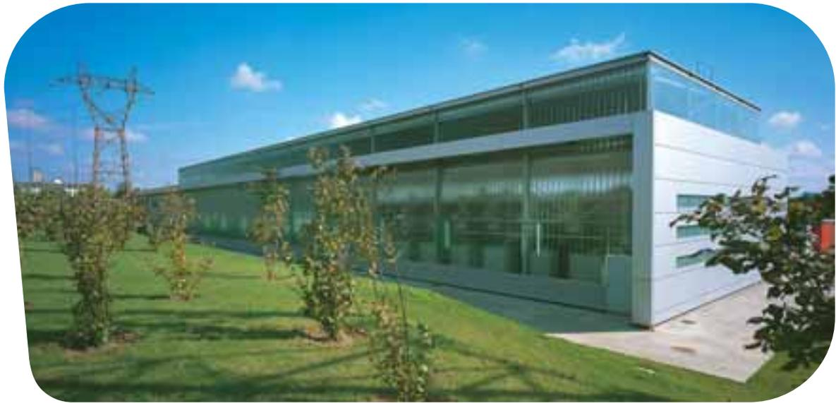
The two long walls of the main rooms (measuring 63 m long, 16 m wide and 9.5 m high) are clad in single layer Pilkington **Profilit™**. The panels are installed to a height of 6.7 m on the south side with no intersection.
