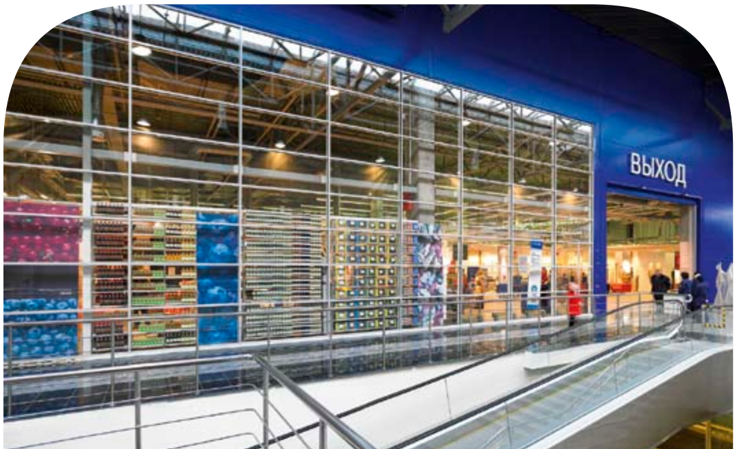
Internal façade with Pilkington Pyrostop ® – IKEA Furniture Store, Moscow (RU)
