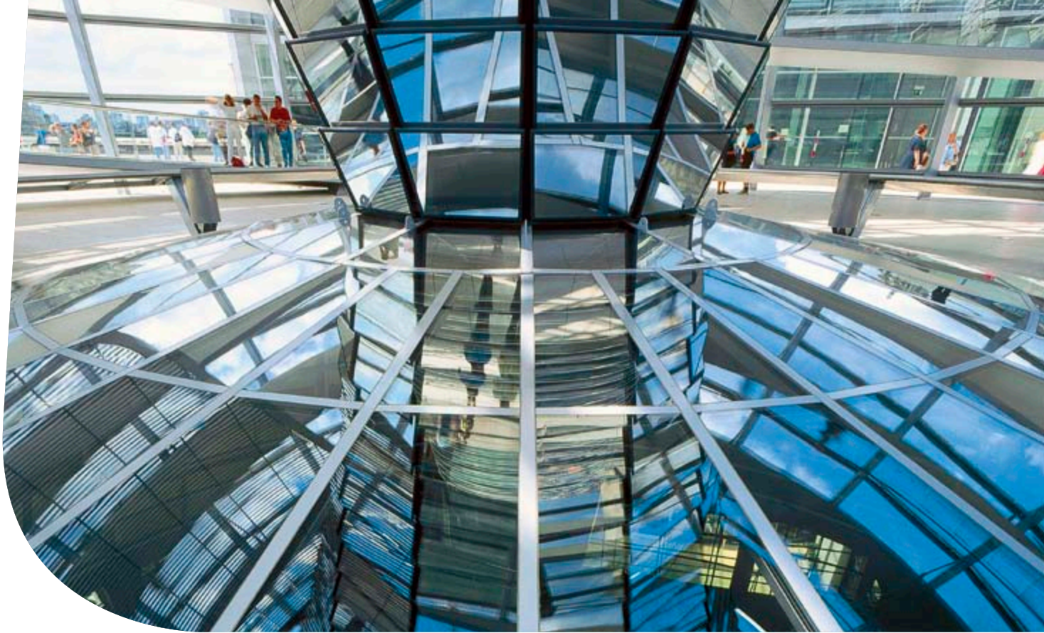
Internal sloped glazing with Pilkington Pyrodur ® installed 1999 – Reichstag, German Parliament, Berlin (DE)
