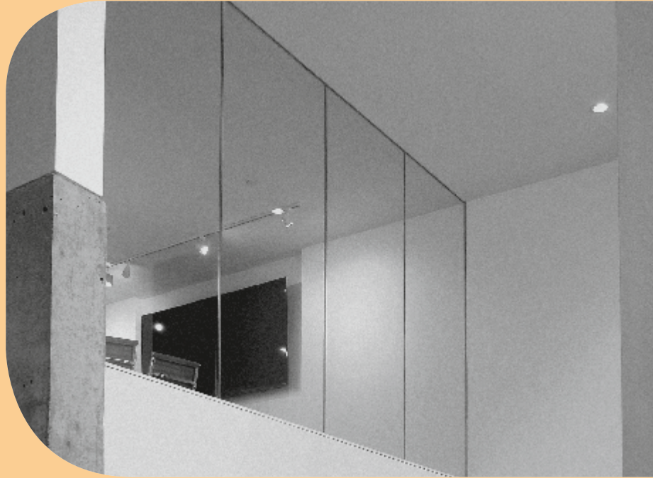
Partition with Pilkington Pyrostop ® Line – Turnstyle Studio, Seattle, WA (US) Image courtesy of Technical Glass Products
