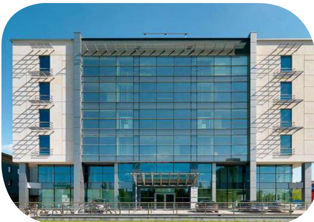
JPBC Business Center, Lublin, Polen. Pilkington Suncool ™ 66/33 T Pilkington Optilam ™ Klar Pilkington Spandrel Glass IGU
