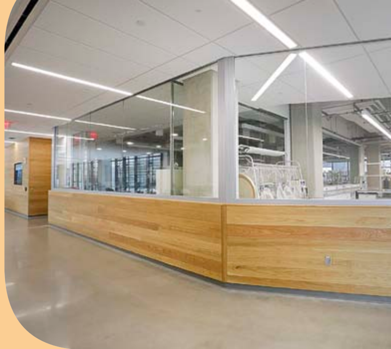
The University of Kansas – Earth, Energy & Environment, Lawrence, KS Fireframes ClearView™ System for EI 60 Image courtesy of Technical Glass Products
