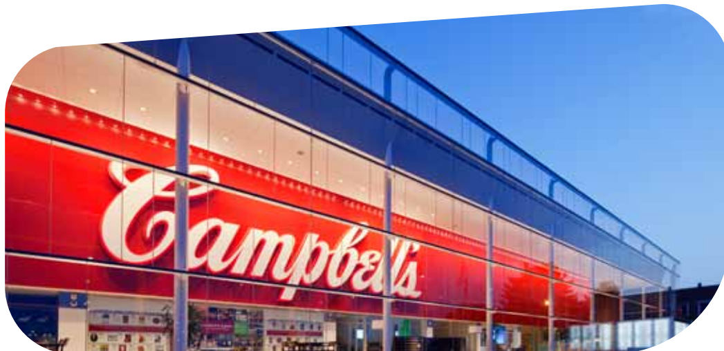
Pilkington Optiwhite™ Campbell's Employee Center, Camden, New Jersey
