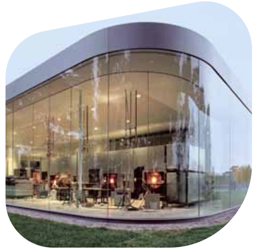
Pilkington Optiwhite™ Glass Pavilion at The Toledo Museum of Art Toledo, Ohio
