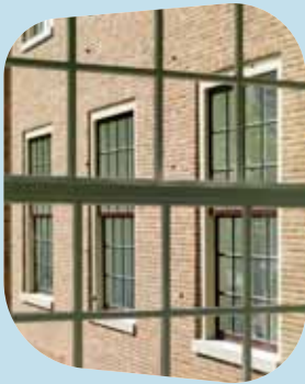
The Hermitage Museum Amsterdam Approximately 900 Pilkington Spacia™ units
